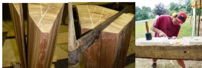
Red Cedar wood is split with an adze to make sure the grain is vertical and runs straight all the way through the blade. Picture on right shows Ed on a Timber Framers Guild bridge building project.
